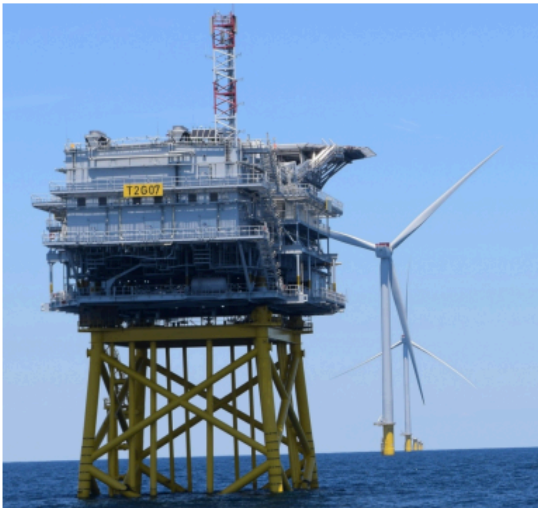
Figure 5: Completed OSS with topside
